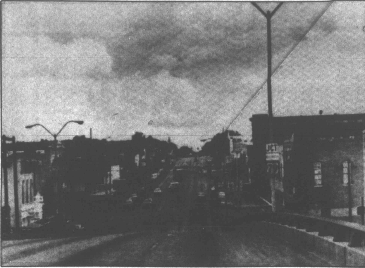
Residents of Taylor, in Central Texas, hope to restore and renovate their downtown area, which has decayed as shopping centers on the "strip" lured the retail trade away. (AP Laserphoto)
