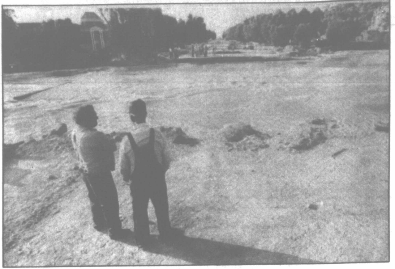
Residents of Deseret, Utah, look at the gap caused when flood waters from a broken dam washed out the bridge that connect the town. The waters are expected to rise even more tonight. (AP Laserphoto)
