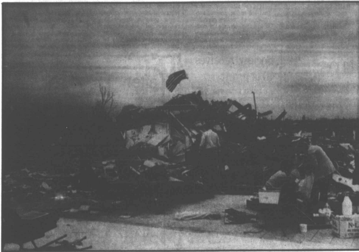
An American flag flies over the rubble that was once the Victory Baptist Church in Paris, Texas April 3, 1982. On April 2, a tornado struck the northeast Texas city, killing 11 and wrecking $50 million worth of damage. The church, one of five destroyed in the storm, and the town have since rebuilt. (AP Laserphoto)
