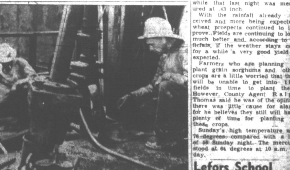
OIL RIG FIRE — Fire struck Well No. C1 on the Jackson lease, 19 miles east of Pampa, near 10:30 a.m. today. Four persons were injured with only one, H. B. Roberson, being admitted to Highland General hospital. His condition was reported "fair" at 1 p.m. today. The others, James Sutt, Charlie Jameson and Rupert Jameson, were given emergency treatment and dismissed. In the above photo, Capt. Paul Skidmore (right) and an unidentified oilman (left) look over the damage on the rig platform. A "good bit" of damage was reported. Cause was believed to have been a pilot light in a trailer house north of the rig. (News Photo)
