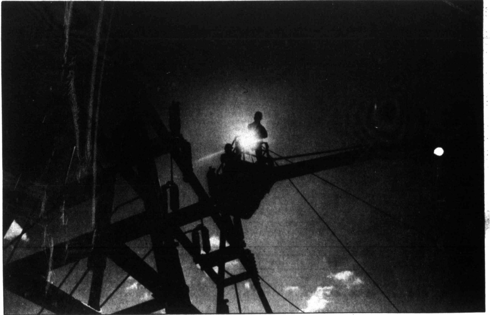
Workmen from SPS are putting the finishing touches on the new power substation on Harvester.
