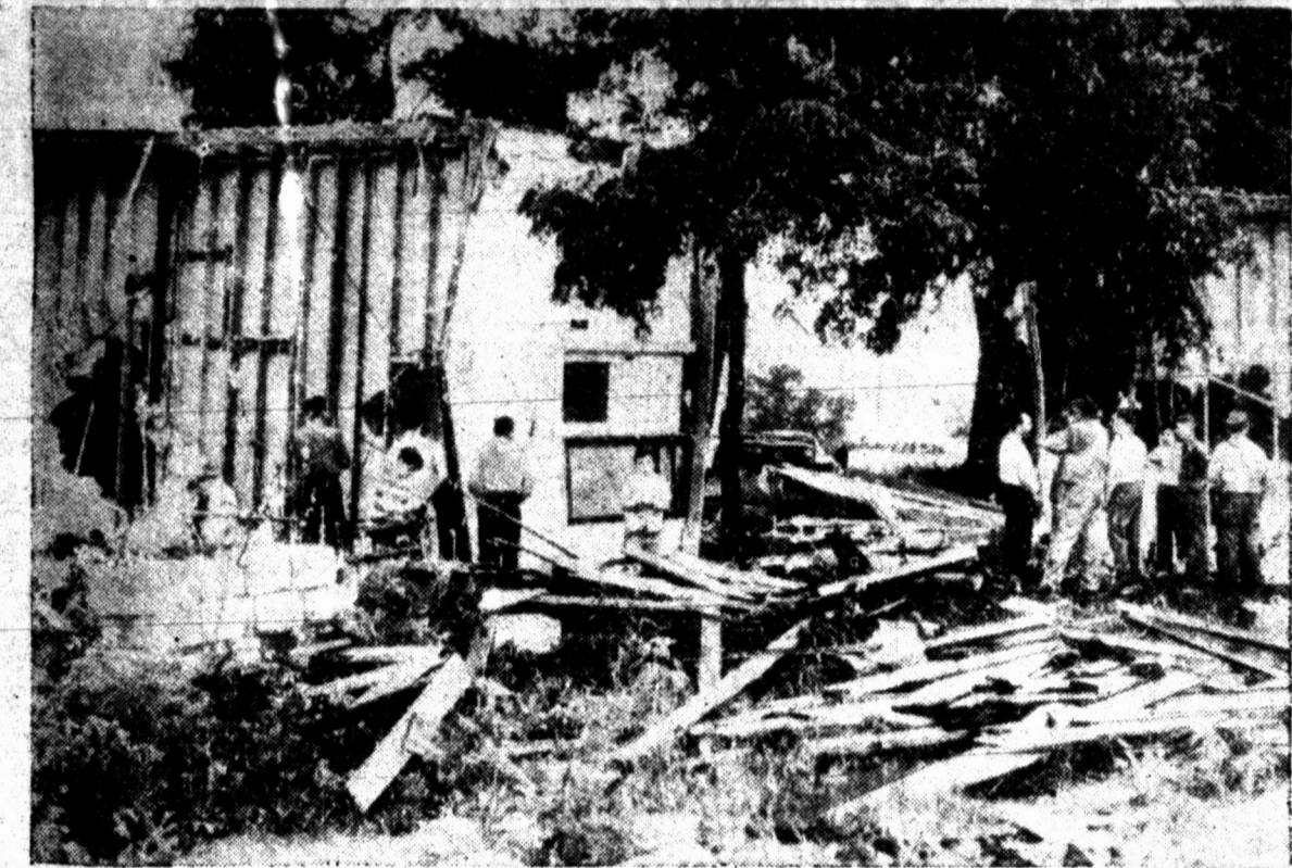
TORNADO SPLITS STUDENT'S HOME IN HALF—University of Illinois student Hugh Robinson, of Cranford, N. J., was taking a shower in his Champaign, Ill., home when a tornado hit 16 blocks of the city and split his house in half. Here curious spectators examine the separate sections.
