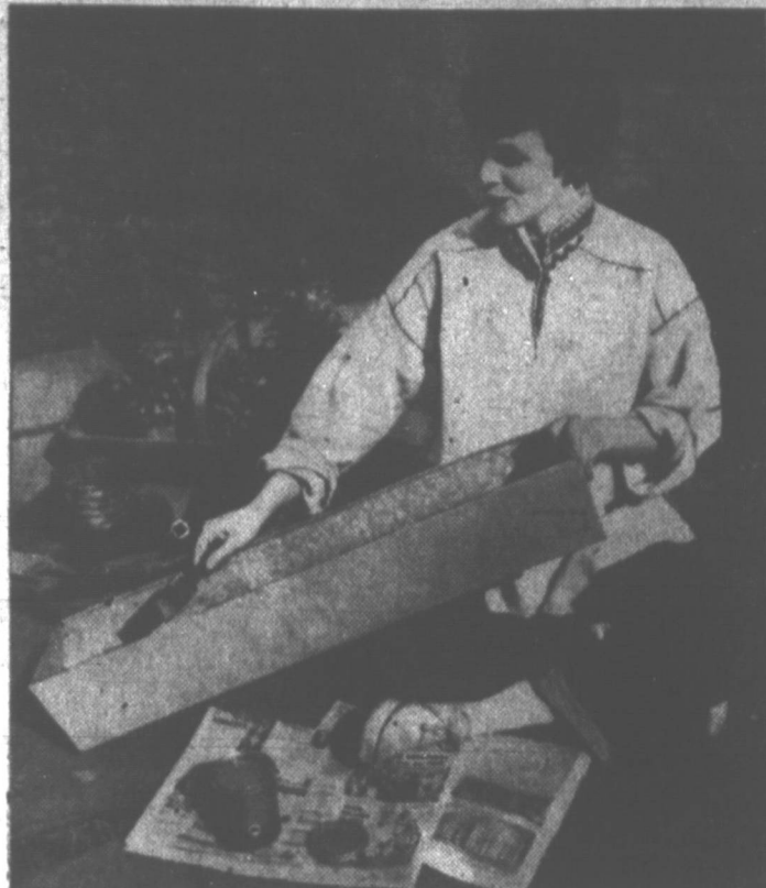
She's painting the inside of a metal planter with liquid neoprene rubber, which protects against rust and rot. It also can be used to skidproof handles of your garden tools, and has numerous other out-of-doors uses.
