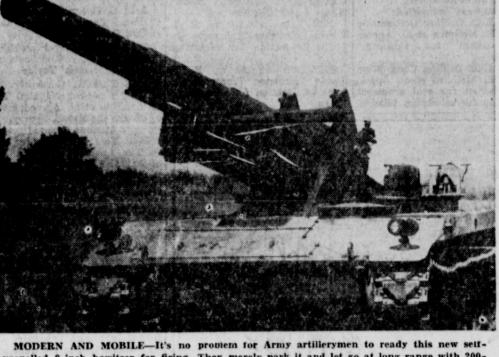
propelled 8-inch howitzer for firing. They merely park it and let go at long range with 200pound shells. The tracked carrier was designed to move at high speed across rugged terrain.
