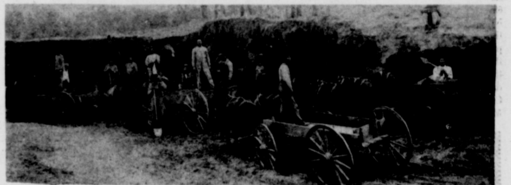
EARLY EASTLAND COUNTY ROAD CONSTRUCTION (location unknown) Photo owned by Mrs. Jack Mace and Ada V. Cox
