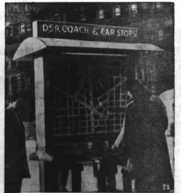
ROBOT BUS FINDER — Pushbutton map in downtown Detroit shows people where to board bus or streetcar. When bus line button is pushed, locator bulb lights on map.
