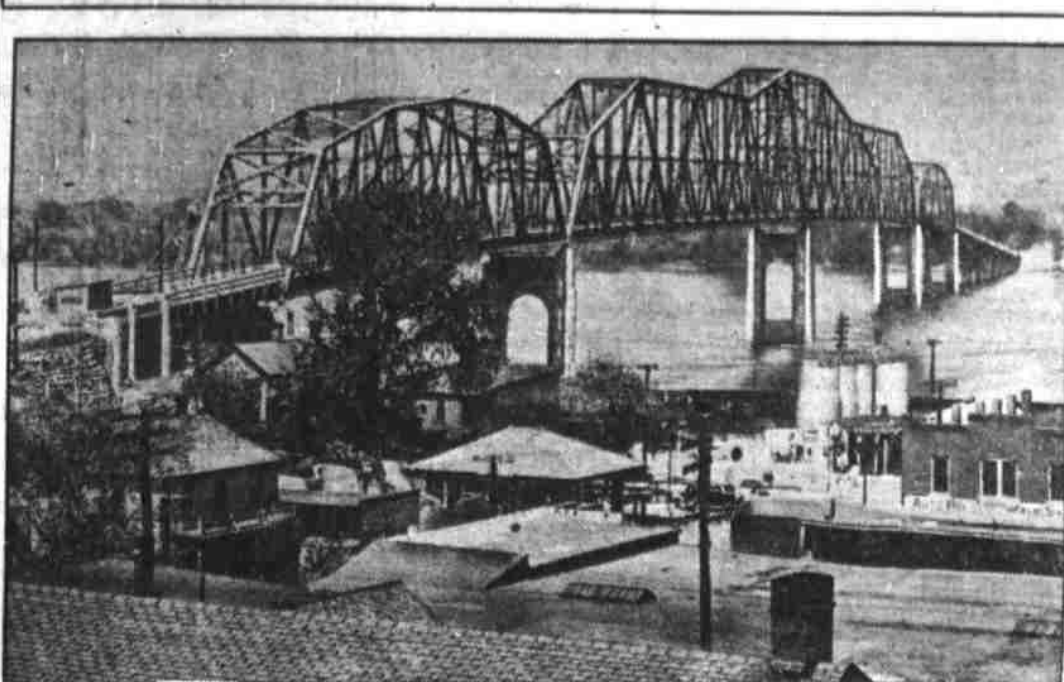
This is the new Mark Twain bridge over the Mississippi river at Hannibal, Mo., to be dedicated September 3 by President Roosevelt on his tour of drouth stricken states. The sloping side of Cardiff Hill, made famous in the stories of "Tom Sawyer" and "Huckleberry Finn," form the west approach of the recently completed span. (Associated Press Photo)
