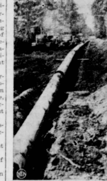
War-time demands for oil in eastern U. S. rushed construction of Plantation Pipeline to carry gasoline from Louisiana to North Carolina. Piece of pipeline is shown being lowered into three-foot trench that hides it from air attack.
