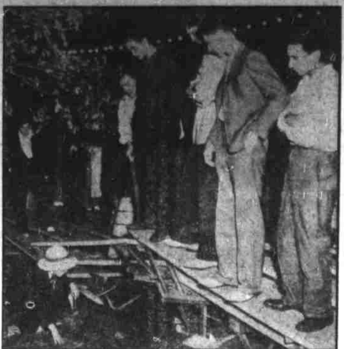
Fifty persons were injured, one seriously, when three crowded spectator stands collapsed at Philadelphia under weight of the hundreds of persons trying to obtain a glimpse of the Mardi Gras parade staged for the amusement of the Democratic national convention delegates. (Associated Press Photo)
