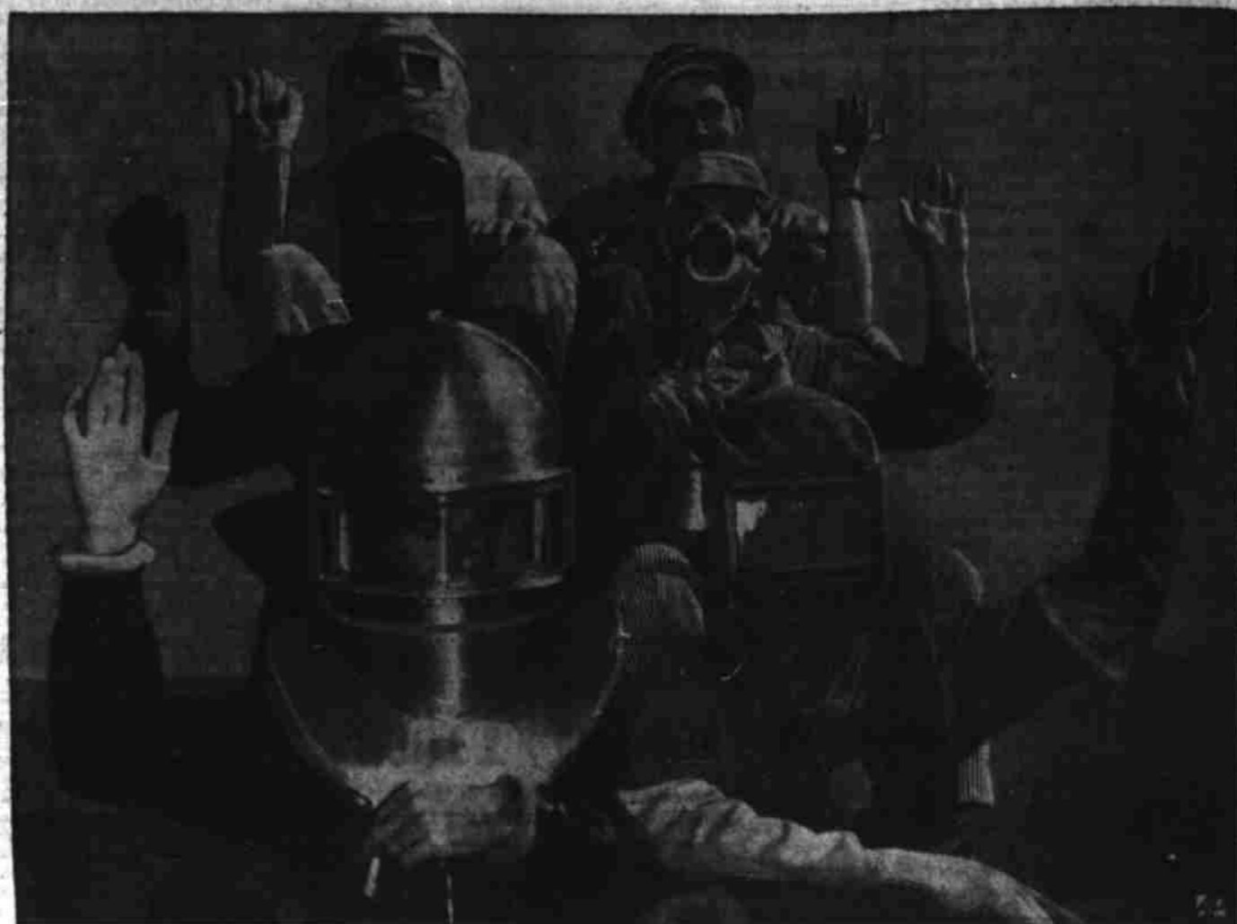
WORKERS IN WAR AGAINST INJURY. —Last accidents result in grave loss of time harmful to defense, workmen don all sorts of protective attire, as did those six in Douglas Aircraft plant at Santa Monica, Cal. To guard his lungs, the spray painter wears a special nose mask; the plant fireman is encased from top to toe in asbestos; welder, sandblaster and "cold-room" research man wear queer headgear and leather garments; man working on high steel wears crash-proof military helmet to deflect dropping bolts.
