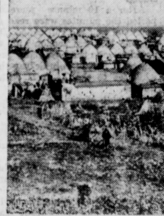
Typical Syrian town features domes for roofs. Construction helps make interiors livable despite intense heat.
