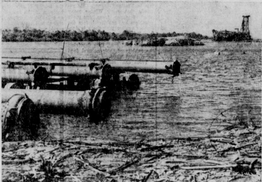
A new link, considered vital to hemisphere defense, is rapidly being formed in "America's lifeline"—the Panama Canal. It is a third set of locks, offering an alternate route in wartime in case of damage to existing locks. Photo above shows Atlantic approach of new locks, with Gatun Lake at left. At right, huge suction dredge is digging out a channel. In many areas army engineers had to level tropical jungle such as appears on far shore.
