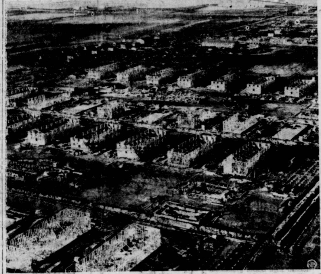
Mushrooming up on the Kansas flats near Fort Riley is this "city"—the army's new cavalry replacement center. Uncle Sam will populate it, too, for the center will house 7000 draft trainees.
