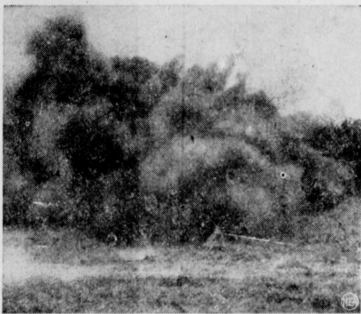
Boom! Hidden in this thick burst of black smoke and powder is the answer to a question that's most important now that an expanding U. S. Army calls for all available materiel: How good is the equipment of World War days? To find out, army engineers blasted an old 7 1/2-ton Renault tank with a 12-pound TNT land mine at Fort Belvoir, Va. Below is what they saw when smoke cleared away.
