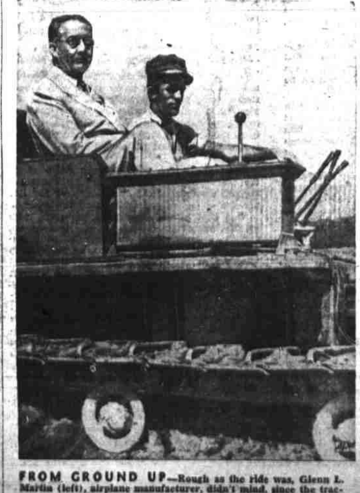
FROM GROUND UP—Rough as the ride was, Glenn L. Martin (left), airplane manufacturer, didn't mind, since the tractor in which he and a workman sit helped break ground for a huge Martin Aircraft Co. addition at Baltimore.
