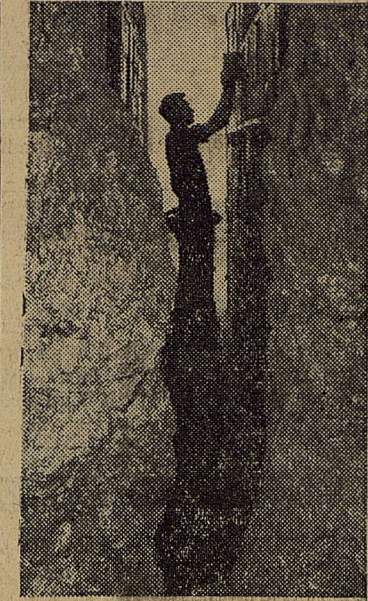
CAVE MAN —George Kendall stores some records in a file 205 feet beneath the ground in a former limestone mine at Butler, Pa. The atomic-age record room has been made for storing records of the Westinghouse Electric Corp. Kendall and three other workers care for some 105,000 file boxes.
