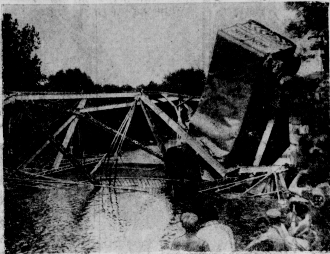
Dumped into Juniata river at Alexandria, Pa., when bridge collapsed, automobile and trailer truck are wedged together in bed of stream. Truck fell on car, smashing it. Occupants of car—Mr. and Mrs. Edwin Kaufman of Sunnyside, N. Y., and young son—died.
