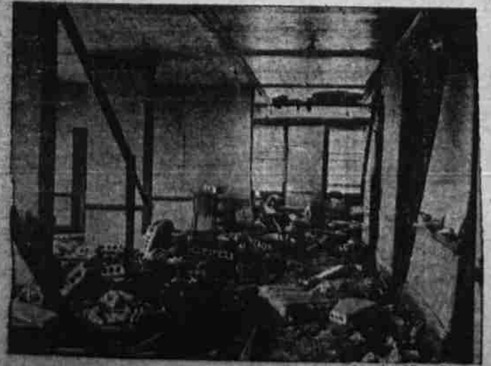
The bomb that wrecked this eighth-floor office of a St. Louis building, detectives believe, was intended for an office one floor below, housing race track news service.
