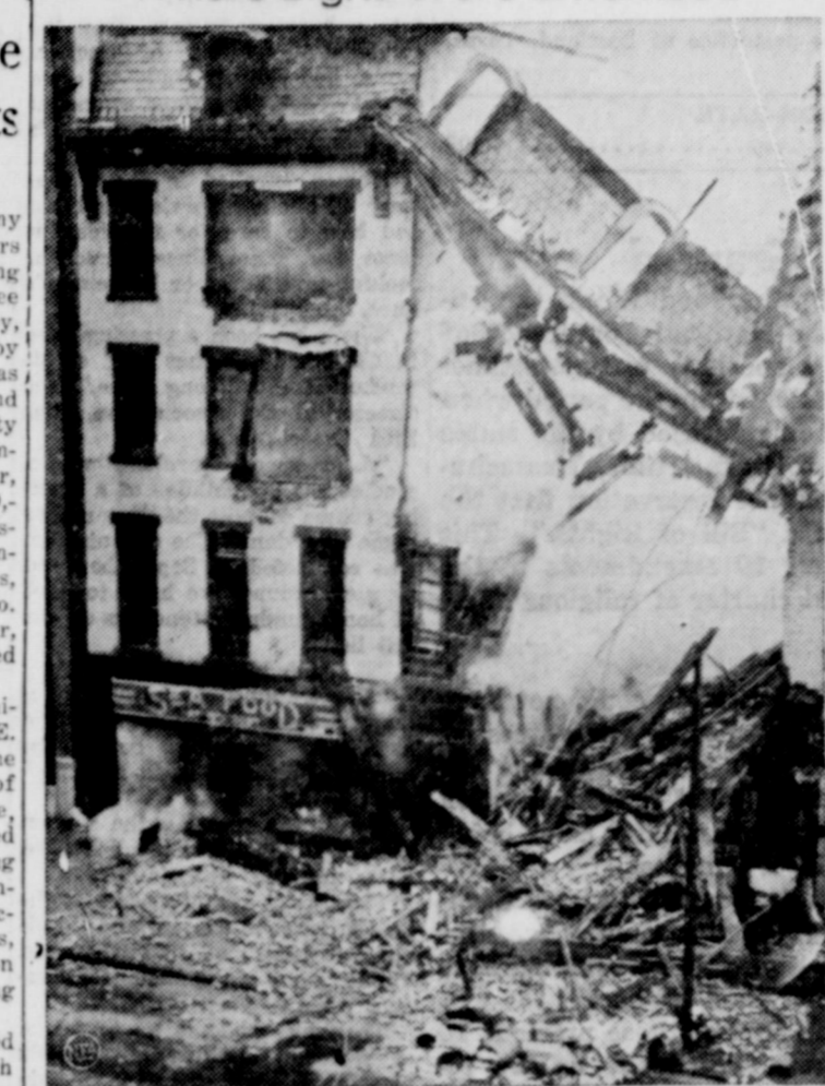
Eight firemen were killed in Syracuse, N. Y., when the roof of this five-story warehouse, pictured at moment of collapse, buried the firefighters beneath tons of debris.
