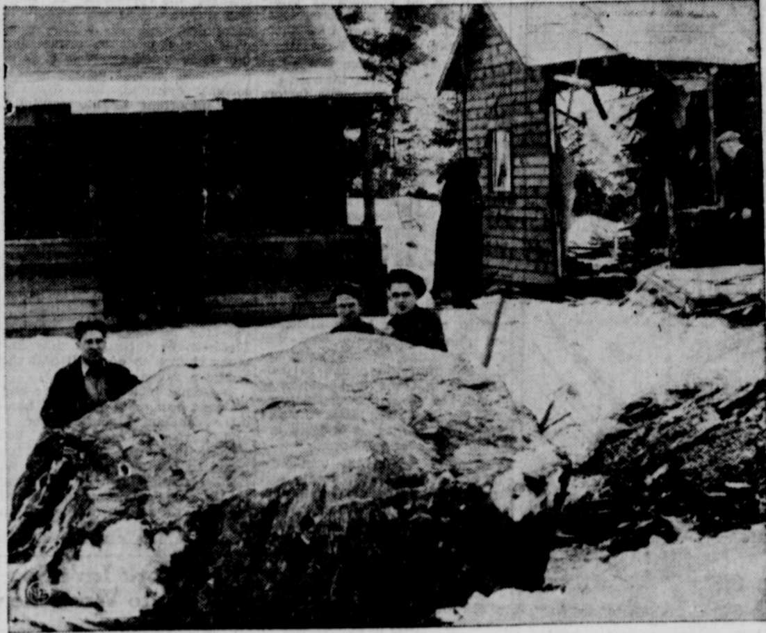
Hurling down a mountainside in Hedley, British Columbia, this great boulder, weighing many tons, smashed through house at right, killing two persons. Homes of 15 families were demolished.
