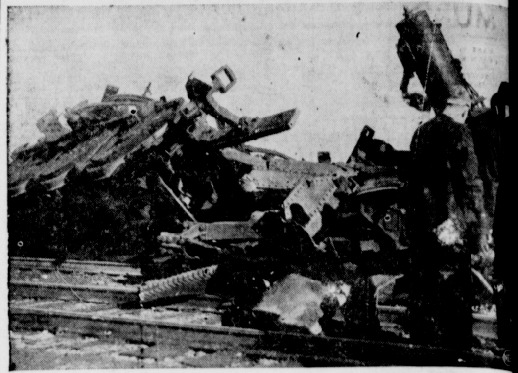
Three men were killed, the boiler was hurled 300 feet, rails were torn up and a great hole dug in the road bed when a railroad locomotive exploded between Elgin and Altona, Ill. The above picture shows the tangle of twisted and broken metal that was left when the locomotive of the Chicago, Milwaukee, St. Paul & Pacific railroad let go with a roar. A fireman, an engineer and a brakeman died in the wreckage.
