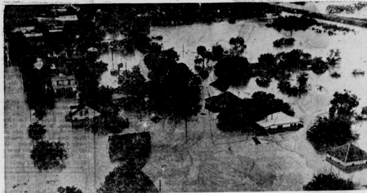
Havoc was created by San Saba's worst flood in history when the San Saba River went out of its banks over the week-end, following heavy rains on the watersheds of the San Saba, Brady Creek and Concho River. Water swirled through the town, reaching almost to second story windows in the residential section, as shown above, while the flood crept into the business section of the town.
