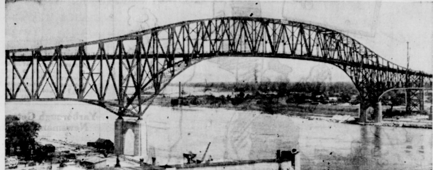
Another steel link binding the United States and Canada will be welded when President Roosevelt goes to Canada in mid-August to dedicate the Blue Water International Bridge pictured above. The bridge, 8000 feet long, and arching 152 feet above the waters of the St. Clair river, connects Port Huron, Mich., with Sarnia, Ont. It cost almost $2,000,000, and commands an impressive view of the junction of Lake Huron with the St. Clair river, a point where teeming lake traffic funnels through the narrow channel. The American and Canadian governments built the respective approaches, and an international commission built the center span. The bridge opens a new fast route between Chicago and Montreal.
