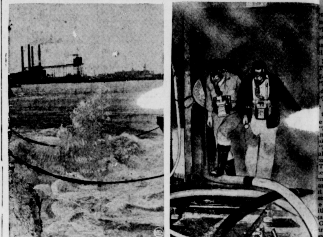
Fire raging in New York's uncompleted $58,000,000 Midtown Tunnel, 90 feet below the East River, was extinguished after 12 hours when the bore of the tunnel was flooded. Firemen, wearing two masks each, are pictured at right above, emerging from the shaft after successful efforts to hose down the flames. Before entering they were tested in compression chambers for ability to stand the tremendous atmospheric pressure. As shown at left, the highly compressed air in the tunnel, displaced by falling rock and clay, forced its way 90 feet upward and shot a geyser 100 feet above the river's surface.
