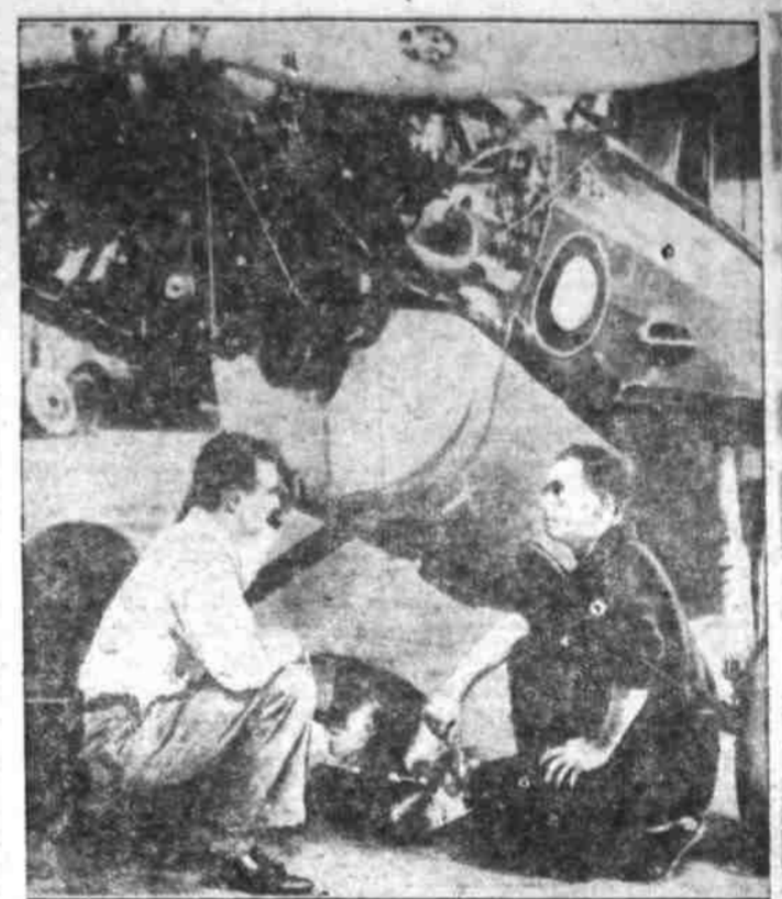
Hugh Herndon, Jr. (left), and Clyde Pangborn, American fliers, shown in Tokyo installing a "chin" tank on their plane a short time before they took off from Samushiro beach, Japan, on flight across the Pacific to the United States. The additional tank holds 50 gallons of gasoline.
