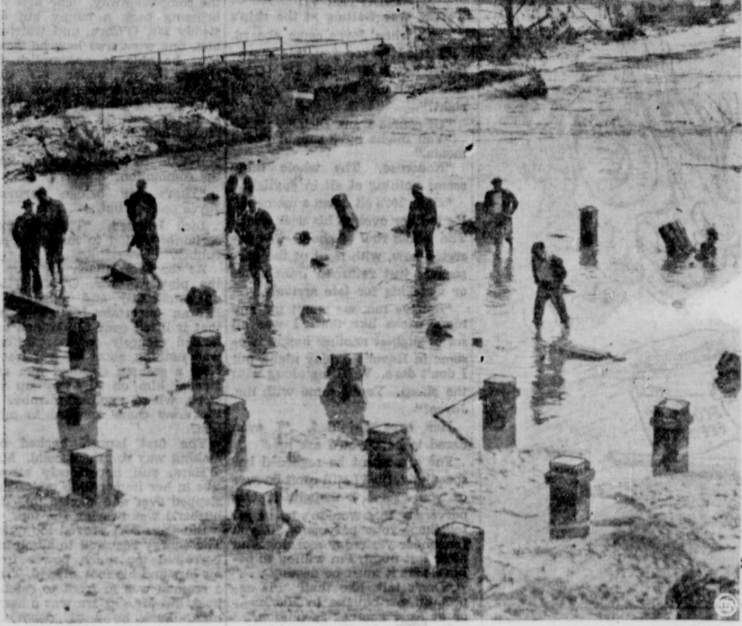
The projecting timbers seen above were all that was left of a house at Whitestone, Ga., where a cloudburst struck like a giant knife, sliced the house cleanly off its foundations, killing 13 people.
