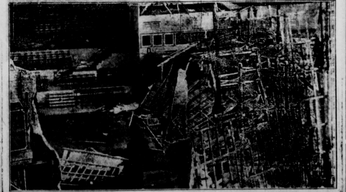
This is what is left of the $250,000 Cavalcade of Texas set at the Texas Centennial Central Exposition at Dallas after a 65-mile-an-hour gale struck the place Monday night. The set was ripped apart, torn and then damaged by fire after lightning struck it. It was one of a number of places in the Centennial grounds that suffered damage, estimated there alone at $100,000. Workmen immediately began rebuilding the Cavalcade set and repairing other damage. The damage at Dallas was estimated at $1,000,000.
