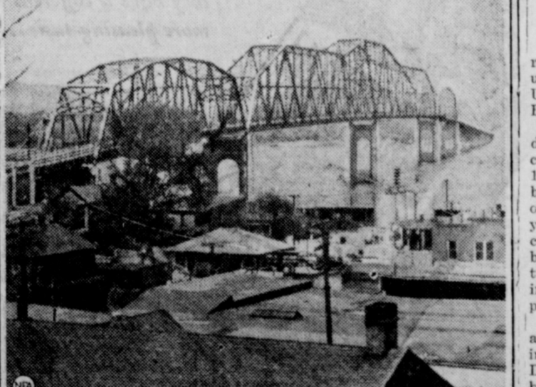
Viewed from Cardiff Hill, famed as a favorite haunt of Tom Sawyer and Huck Finn, this new Mark Twain Memorial Bridge, spanning the Mississippi at Hannibal, Mo., will soon be dedicated by President Roosevelt. Centennial celebration of the birth of Hannibal's most illustrious son was held last year, opened by lighting of a beacon in the Mark Twain Memorial Lighthouse on Cardiff Hill.
