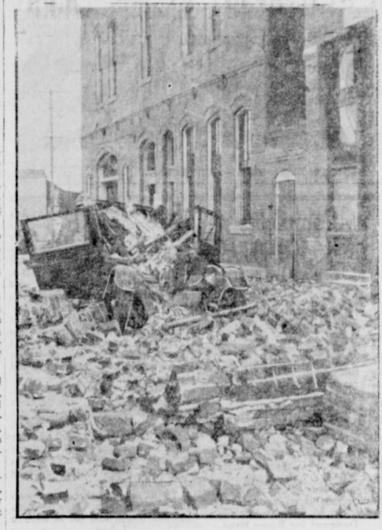
Size of the reconstruction task facing Helena is indicated by this picture, a scene of ruin along one of the capital's main streets, damaged heavily by the recurrent quakes.
