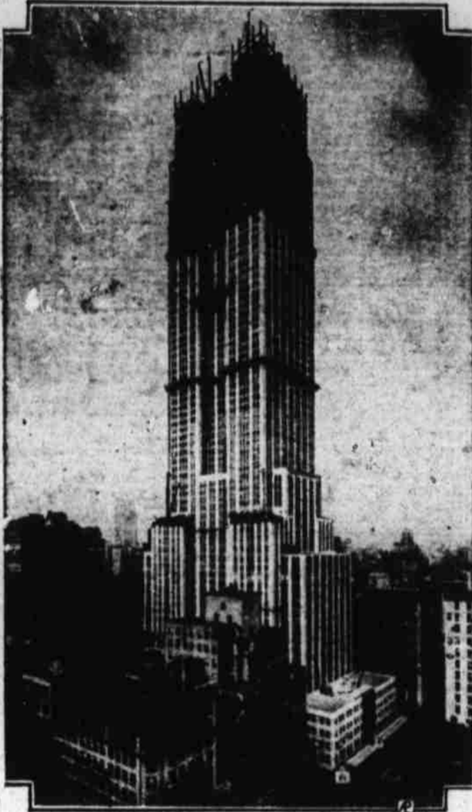
This unusual view of the new Empire State building in New York shows the entire structure. It will be the world's tallest building when the observation mast is added.
