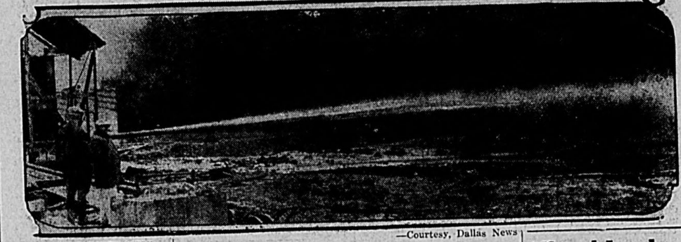
The Hunt No. 1, nine miles east of Eastland in the famous Merriman area, is shown making a flow. The well is estimated at 165 barrels of oil and 1,000,000 cubic feet of gas a day. It was drilled by Col. Robert D. Gordon.
