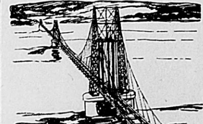
The new 1,760-foot suspension bridge that will carry a Lone Star pipe line over the Red River.
