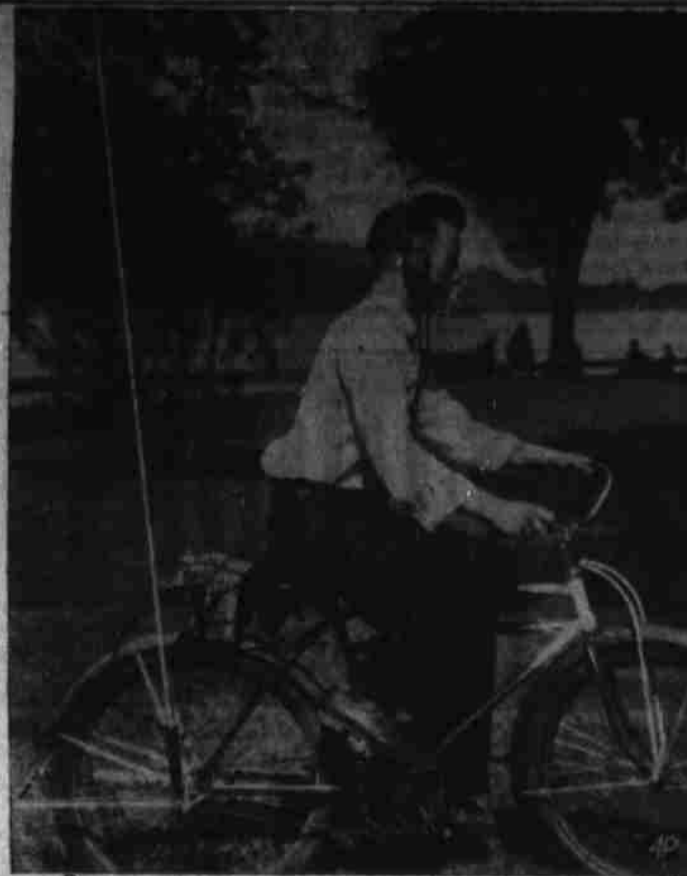
HE SHALL HAVE MUSIC wherever he goes, decided Maurice Reutter, a young radio engineer at Winona, Minn. In his spare time he invented this portable bicycle radio set, complete with earphones for the rider, and an aerial.
