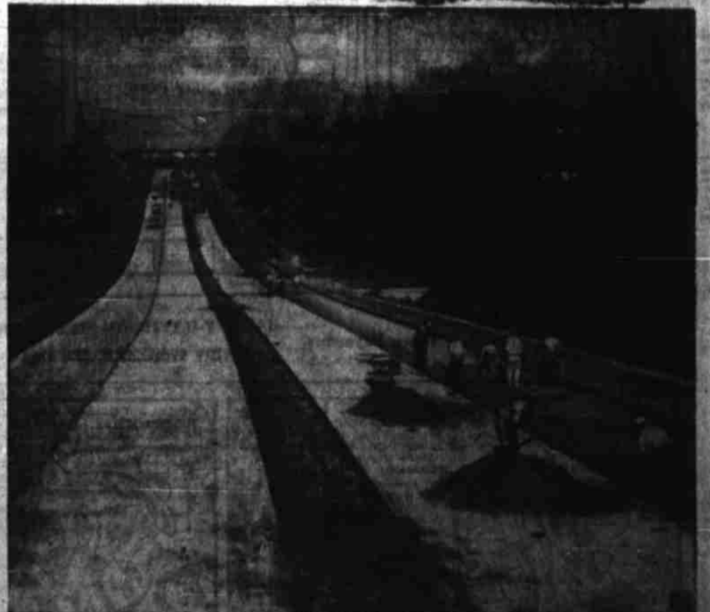
FOUR LANES IN PUERTO RICO —Workmen finish first stretch of $2,200,000 four-lane highway connecting Rio Piedras and Caparra, part of $38,000,000 program on the island.
