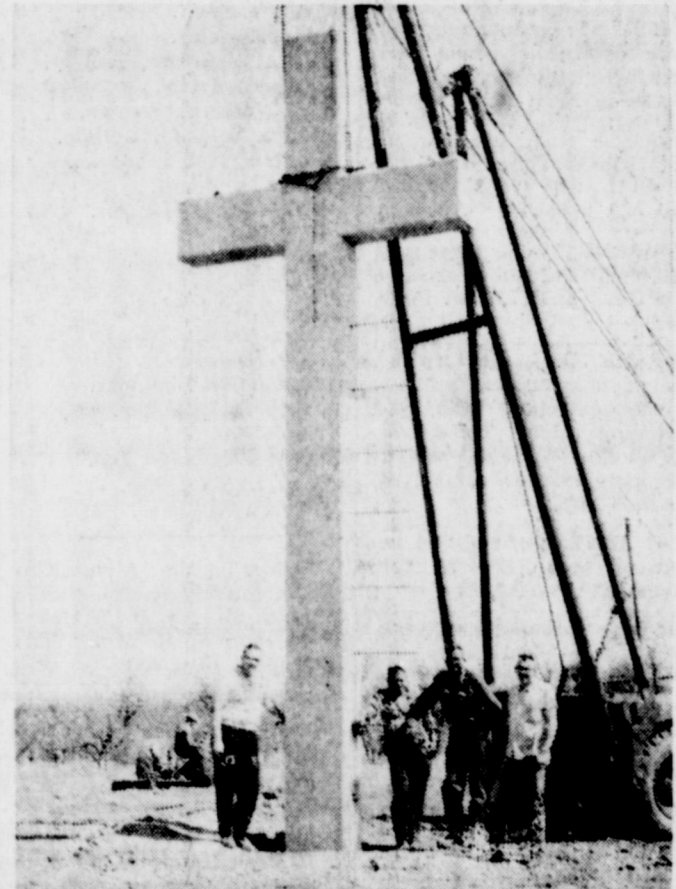
MONUMENT IN PLACE — Appropriate for the season is the erection of this monument at Camp Inspiration, west of town. Shown are Clyde Caselton, Shorty Hibbs, Ralph Taylor and Darrell Basham. The four men put into place the 32 feet high, 15,000-pound cross, made of steel and concrete, at the Church of God Encampment grounds. Dedication will be held at a meet to be held at the camp soon. (Photo by Lloyd)
