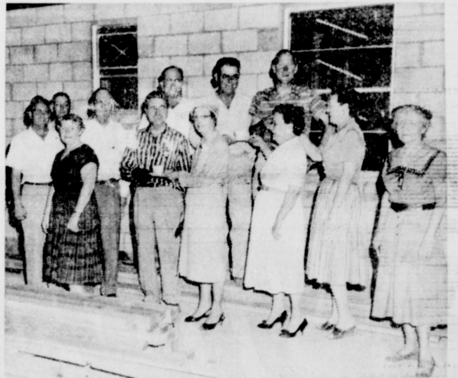
BUILDERS AT WORK — Mr. Hood King, center in stripe shirt accepting a cup of coffee, as Eastland Memorial Hospital was being built by volunteer help. He served as a member of the hospital's first board.
