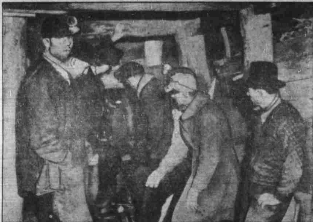
This caved in tunnel, part of a clay pit near Golden, Colo., held three miners prisoners for 18 hours while fellow workers sought to rescue them. In the extreme background W. J. Foreman, one of the entombed men, can be seen crawling to safety after the rescue crew holed through the debris. The others followed him. (Associated Press Photo)
