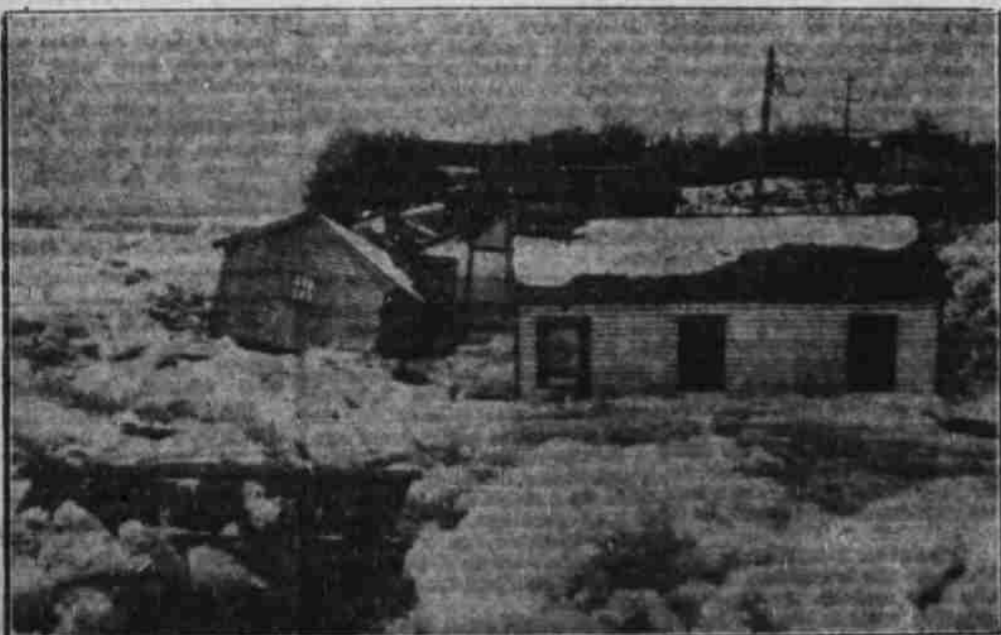
Cottages which line the lower gorge of the Niagara river from Lewiston, N. Y., to its mouth were crushed by the dozen by the great ice jam which filled the gorge from bank to bank. The river was more than 25 feet above normal level. (Associated Press Photo)
