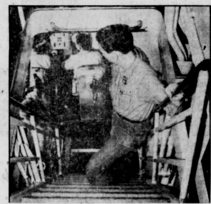
SAILORS GO "DOWNSTAIRS"—They do, if they're assigned to the Nautilus, Uncle Sam's first submarine powered by atomic fuel. Old salts shudder at the substitution of "downstairs" for "below," but the term is appropriate when applied to the nine-step stairway leading from conning tower to diving control compartment.
