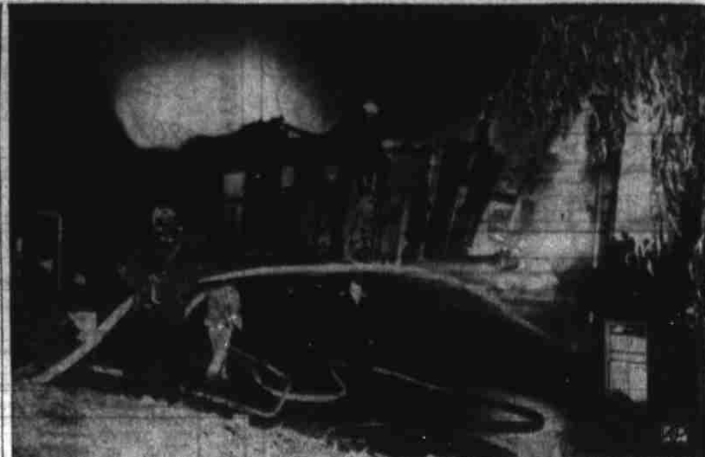
FIRE DESTROYS AEC INSTALLATION —Firemen throw a weak stream of water on the burning Atomic Energy Commission's administration building near the University of California's giant $3,000,000 cyclotron in Berkeley. The building was completely destroyed, but firemen kept the fire from spreading to other structures on the heavily guarded installation. (AP Wirephoto).
