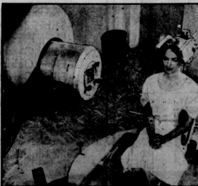
HEAVY ARTILLERY —Big gun in the war against cancer is this six-million-volt linear electron accelerator, recently unveiled at California's Stanford University. Model sits in adjustable, revolving chair which positions a patient in front of gun's muzzle. Generation and projection of high energy X-rays for treatment of deep seated cancer is controlled from outside the lead-lined room. The $300,000 machine was built by Stanford scientists under grants from the American Cancer Society and the United States Public Health Service.
