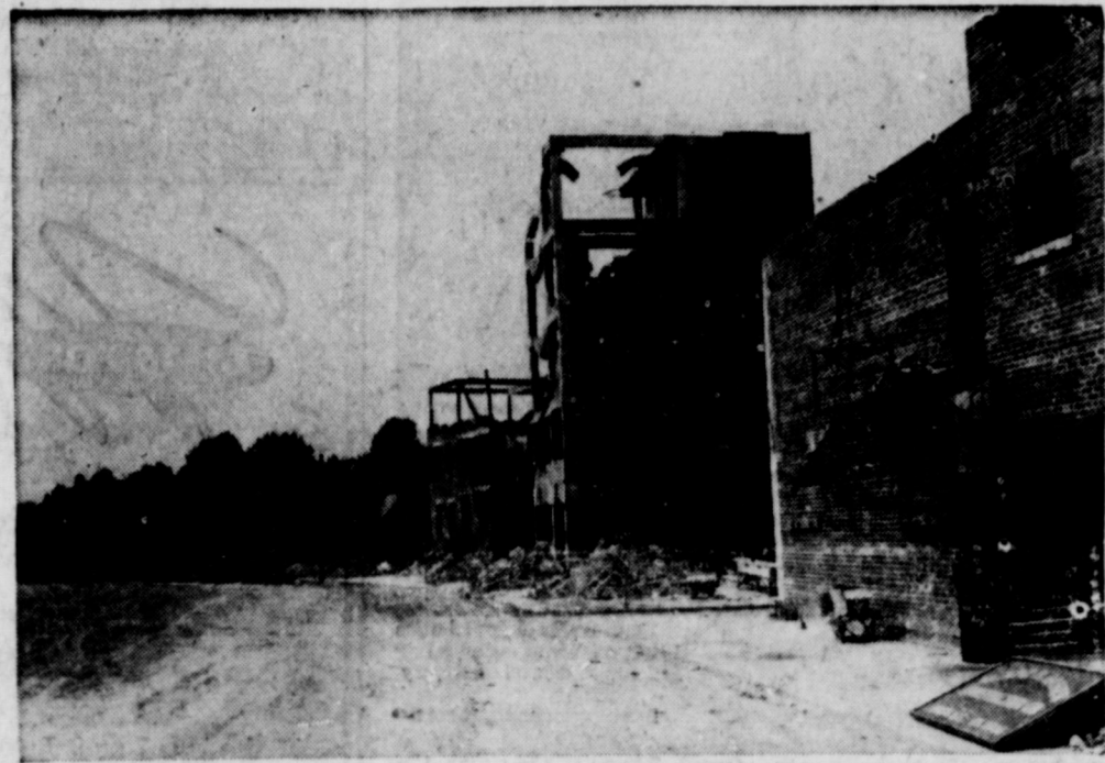
FAMED 'RESCUE STREET' of the Federal Civil Defense Administration's Olney, Md., rescue school, a $200,000 collection of carefully-designed ruins similar to the various structures civil defense rescue workers would face back home in extricable victims of bombings. Up to 70 students are checked out on the built-in obstacles during each week or two-week course.
