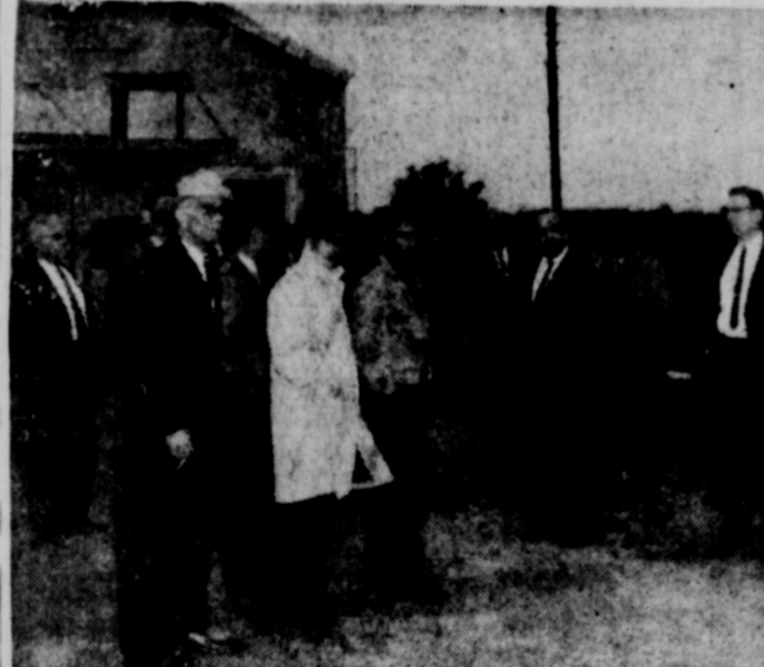
COUNTIANS INSPECT INDUSTRIAL SITES
