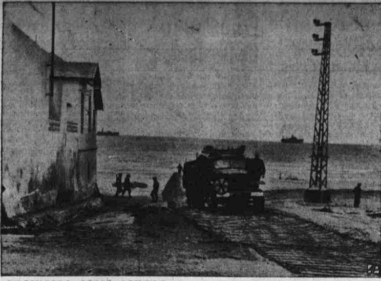
ENGINEERS COME ASHORE—On a road of steel wire and frame work built on the North African sands by U. S. Army Engineers, a 18-wheel truck comes ashore.
