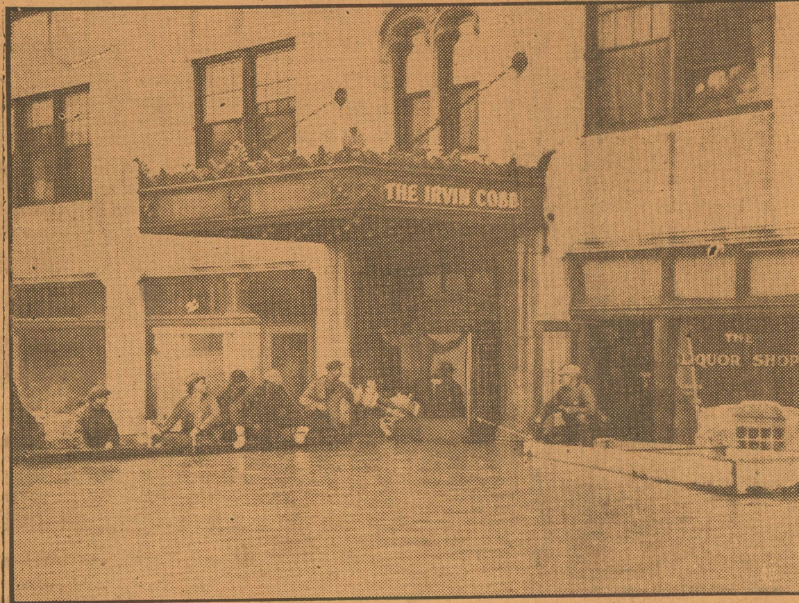
One man holds the wide front doors open and another steers the outboard motorboat right into the lobby of the Irvin Cobb Hotel at Paducah, Ky. Though the first floor was flooded, the hotel was made a concentration point for refugees because it is on one of the town's highest points. Fourteen were reported drowned, most of the 25,000 residents had fled, and troops ruled under martial law.
