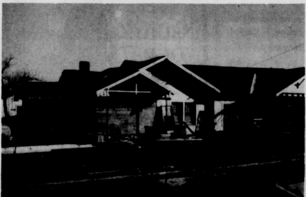
Bakker Funeral Home Soon To Be Completed Photo by H.D. Alsop
